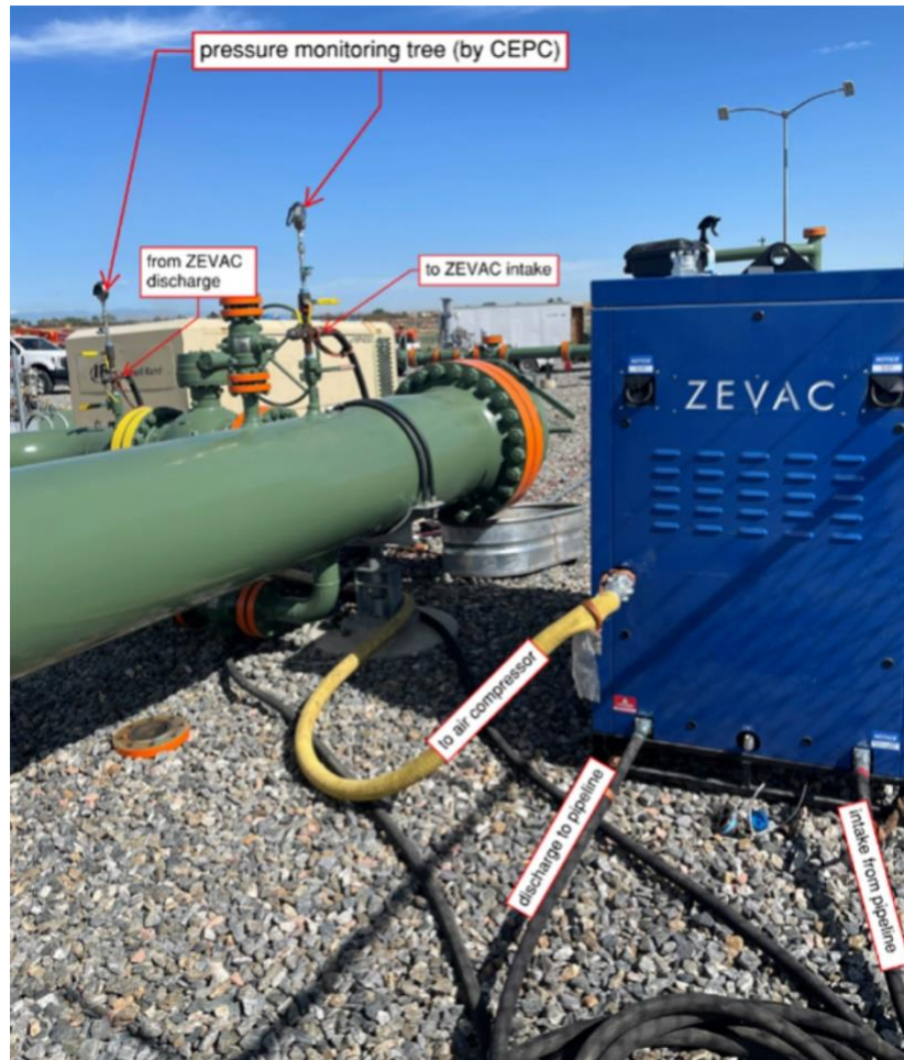
Figure 57: ZEVAC drawdown setup at receiver
