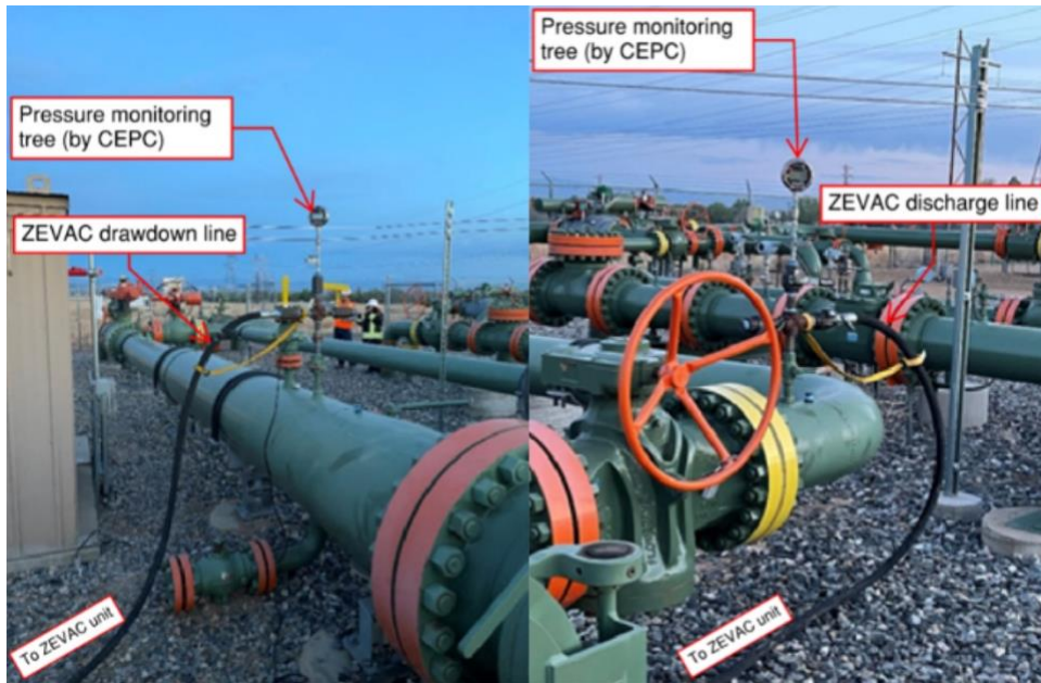
Figure 56: ZEVAC drawdown setup at launcher
