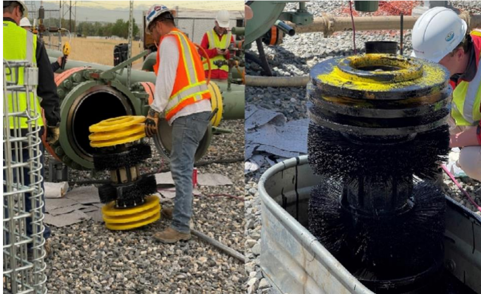
Figure 53: Cleaning "Pig" before and after operation
