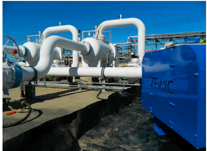
Figure 4: ZEVAC pumping Y-grade from a filter-separator at a pipeline facility
