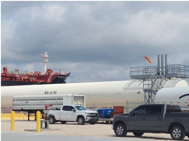
Figure 3: ZEVAC performing liquid butane bullet tank emptying in a port
